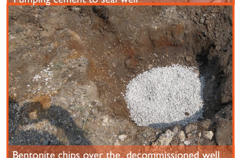
Bentonite chips over the decommissioned well
