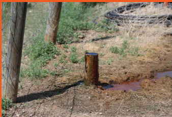
Flowing abandoned well
