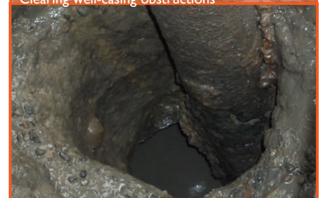
Restoring casing integrity prior to cementing well
