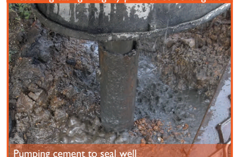
Pumping cement to seal well
