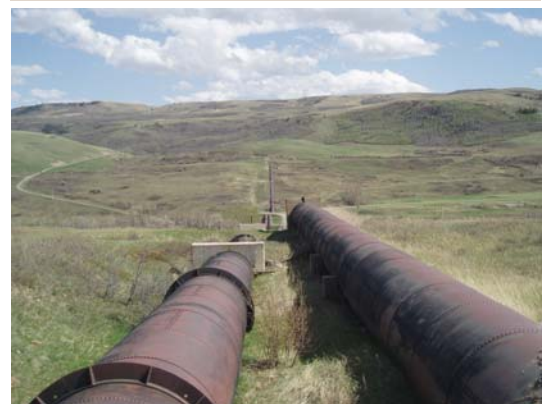
Siphon, constructed in 1917, that delivers water to the Milk River from the St. Mary River. Photo: S. Riemersma
